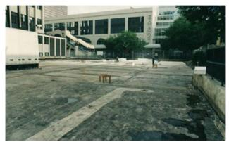
GeoSpec lightweight fill material was used over an underground parking garage as part of the renovation to the Calgary Court of Queens Bench building. The load induced on the underground parking structure due to surface landscaping needed be reduced. A portion of the soil fill material above the garage was replaced with GeoSpec lightweight fill material and the landscaping was completed.
